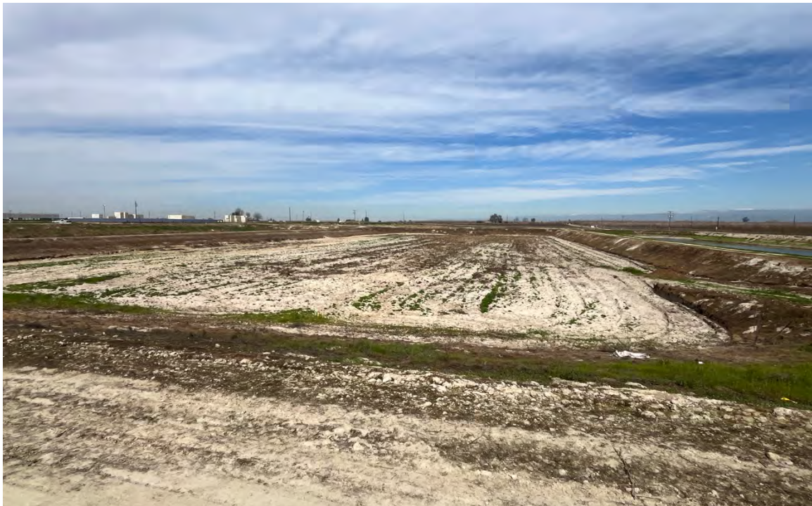
Figure 8. Photograph of the wastewater treatment plant, looking north, showing a road, ruderal vegetation, and a recently disced storage pond.
