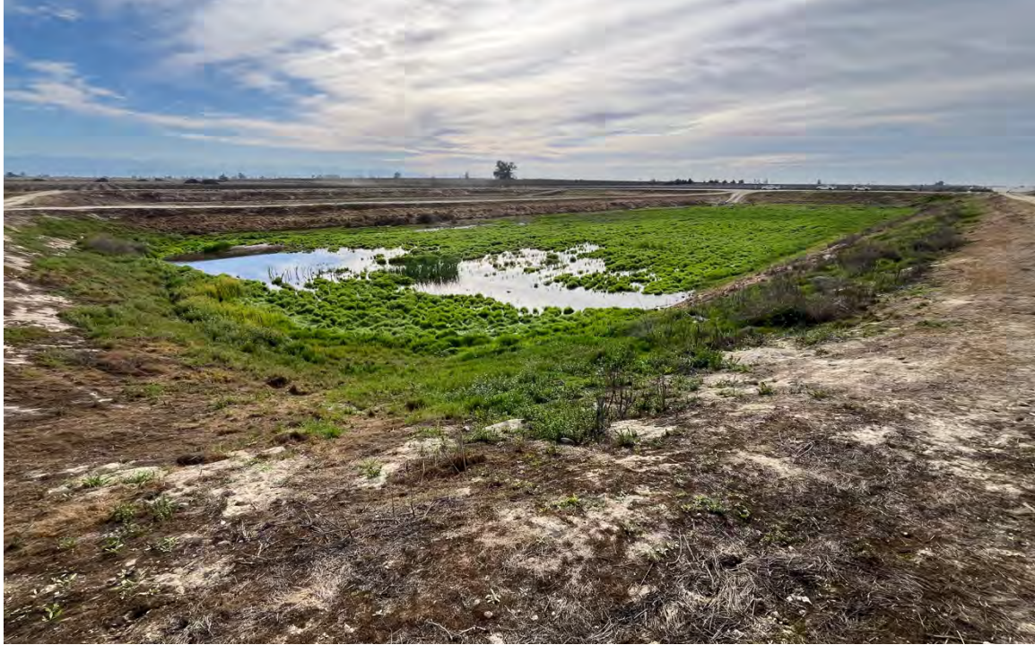
Figure 9. Photograph of the wastewater treatment plant, looking southeast, showing a partially inundated storage pond, ruderal vegetation, and roads.
