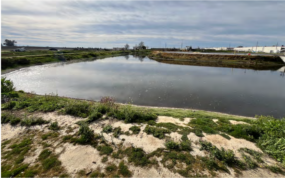
Figure 7. Photograph of the wastewater treatment plant, looking south, showing an effluent pond and ruderal vegetation with facility infrastructure in the background.
